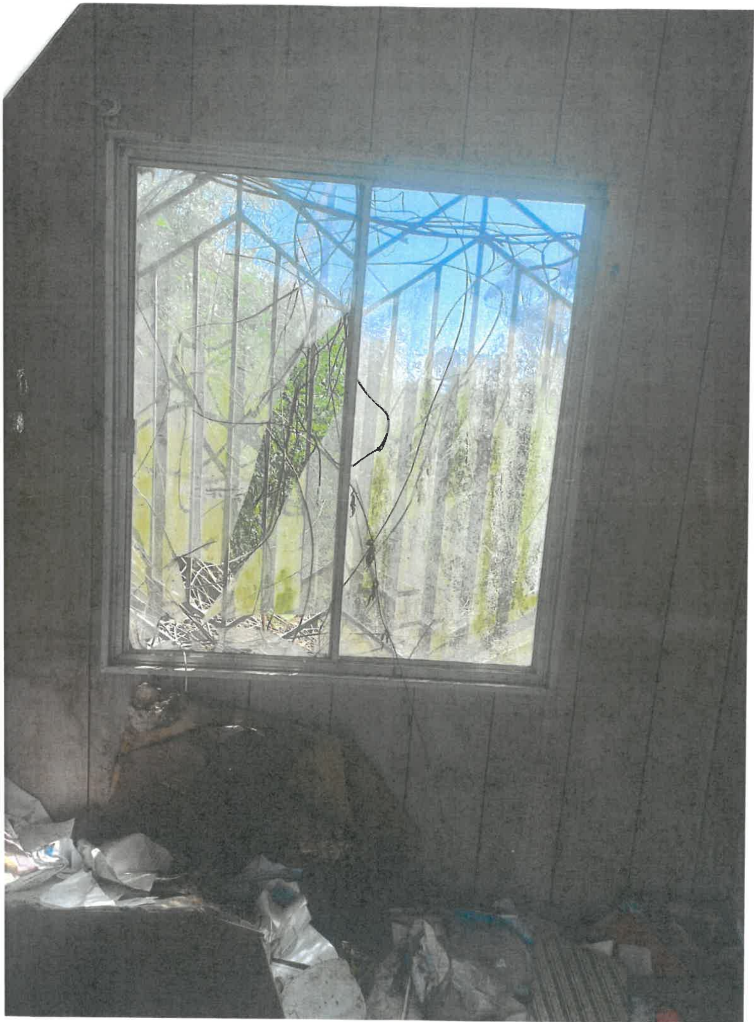
Broken window replacement
