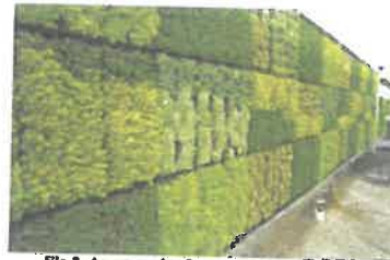
Fig.2. An example of a green gabion basket.
