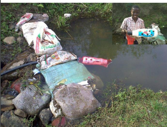
Fig. 2.5 An initial temporary weir made with sand bags. A crude filter made from a plastic bottle (inset top right) was enclosed in an orange bag and fitted to the opening of the siphon pipe.
