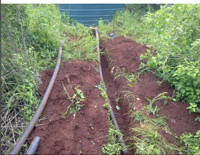
Fig. 5.3 Showing the piping connection to a JoJo tank uphill from the ram pump and roughly about 300m from it. This tank provided water head pressure close to 1.5 bars at the land where irrigation was supplied.
