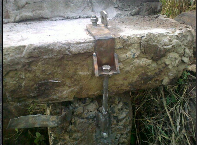
Fig. 4.2 Showing how the weir lintel was attached to a lateral strut by custom made stainless steel anchors bolted to the weir lintel and the strut on the upstream side.
