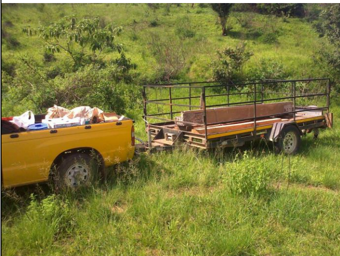
Fig. 3.3 Commencement of construction of a weir by transport of a large concrete lintel salvaged from a demolished building at Cedara to the ram pump site on a trailer.
