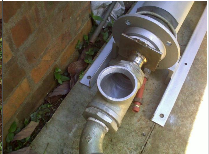
Fig. 1.4 Ram pump assembled except for the impulse valve to screw into the large threaded T (center). Barely visible at the top of the outer nipple of the fitting screwed into the pressure vessel is a sniffer valve comprising a hole with a slotted machine screw in it.
