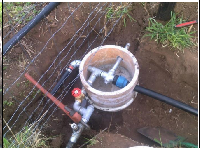
Fig. 5.6 The pipe couplings at the upper centre of the land. The large pipe at the right connects to the pipe couplings shown in Fig. 5.5 The pipe to which the pipe wrench is attached went down to irrigation connection points along the fence between adjacent lands.
