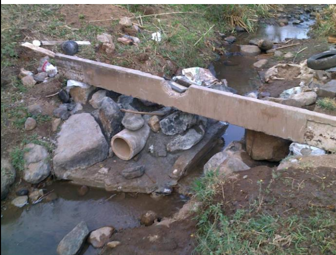
Fig. 4.5 Showing progress with weir concreting from the downstream side with the sluice pipe already concreted in.
