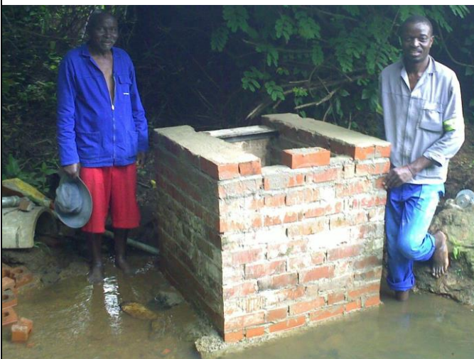
Fig. 2.3 Mini pump house to shield the ram pump, just after completion of the brick laying by 2 locals. The foundation should have been excavated to solid rock and its height should have been much lower because eventually a massive flood ripped the whole thing out.
