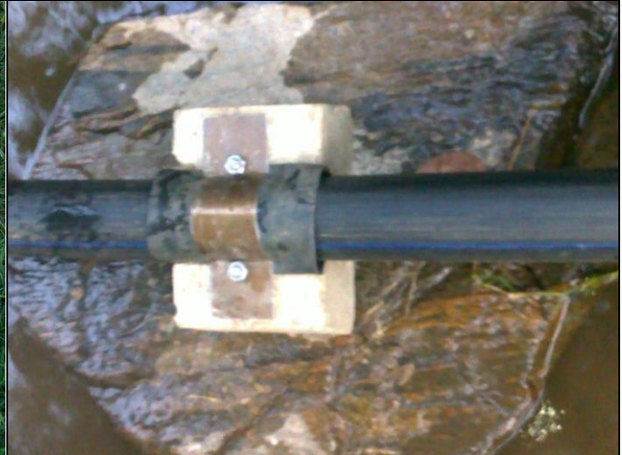
Fig. 3.2 An illustration of a siphon pipe clamp that was mounted on a rock in the river. The outer stainless steel flange was held down by nuts on two threaded rods that were embedded into the rock.
