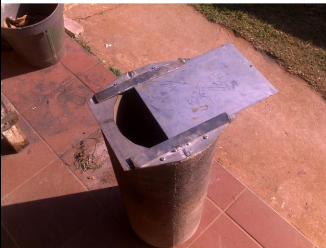
Fig. 4.3 A custom-made weir sluice pipe made from a stainless steel flange screwed to the end of a concrete pipe that had slots either side for a plate to slide. This sluice pipe functioned amazingly well.
