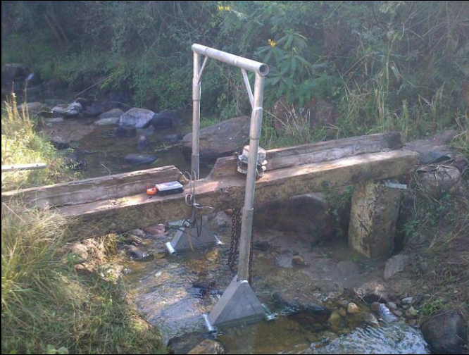
Fig. 4.1 Showing the weir's lintel after lowering into position on its two lateral concrete struts. The steel scaffold shown here was used to position the lintel and it was made by Michael Relihan.
