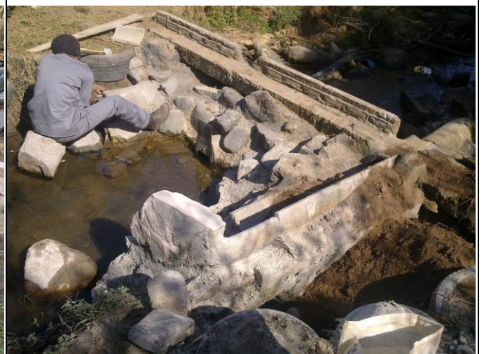
Fig. 4.6 Late stages of weir concreting. A stainless steel pipe was fitted through the weir at the location where the helper is working for connection to the siphon tube.
