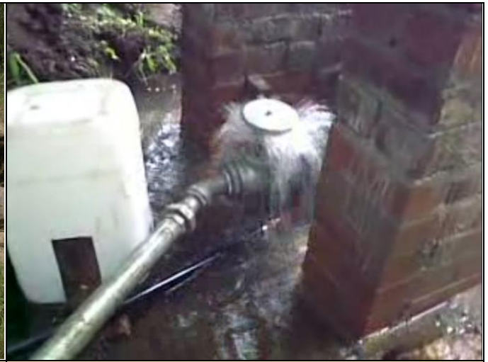
Fig. 5.2 A cell phone video frame of the operating ramp pump at an early installation stage. Its operation was improved by removing the disk weight from the impulse valve which had springs installed on its shaft instead.
