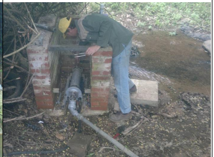
Fig. 2.4 Michael Relihan attending to the ram pump after installation. In the foreground going right is a 1.5 inch NB drive pipe that connected to a stand pipe on the bank of the river. A small black plastic pipe (lower left) is the ram pump output pipe going up the hill.
