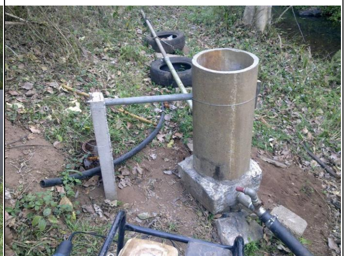
Fig. 2.6 The stand pipe made from concrete pipe that connected the siphon pipe (bottom right) to the drive pipe for the ram pump (background). Stabilized by cable attachment to a concrete stake.
