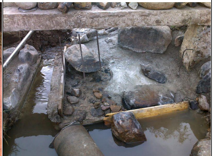
Fig. 4.4 Showing concreting of the weir. The entire base was excavated down to bed rock and concreted in sections allowing flow of the river at each side of it prior to concreting in the weir sluice pipe.
