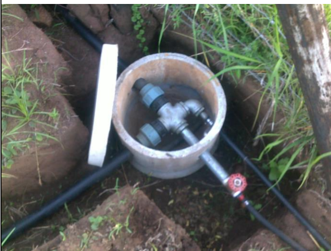
Fig. 5.5 The pipe couplings between the ram pump (shown far lower right), the JoJo tank (shown upper left) and the irrigation line to the land (shown lower left). A second infeed pipe from the river was also installed (with tap) to which a petrol pump could be connected.
