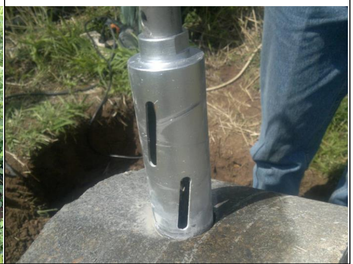
Fig. 5.4 Showing how a diamond coring bit fitted to a heavy duty drill was used to make holes into concrete pipe segments for protecting pipe couplings.
