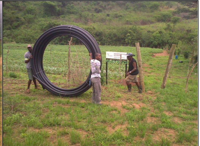
Fig. 2.2 The site at Vulamehlo to which the HDPE piping was delivered. Background is an area planted to potatoes as a Potatoes SA transformation project. This piping was used for the siphon pipe in the river (below).
