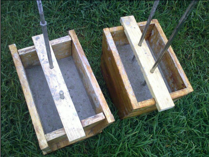
Fig. 3.1 Cement castings of clamp bases made for anchoring the siphon pipe to rocks in the river.
