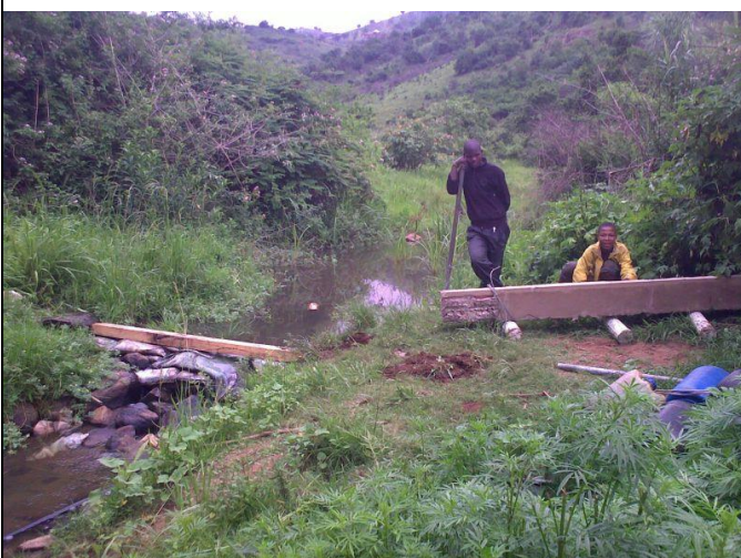
Fig. 3.5 Illustration of the weir's lintel adjacent to where it would be installed on the river. Local youth attending.
