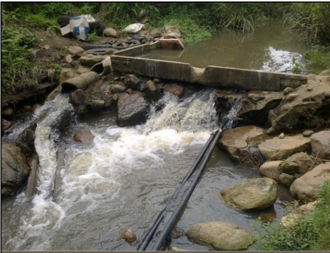
Fig. 5.1 The weir after completion of concreting. To improve flow down to the stand pipe two siphon pipes were installed as shown.
