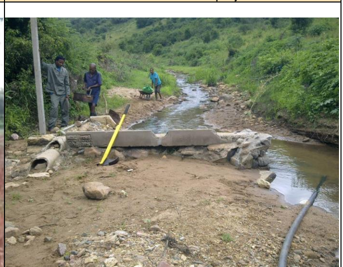
Fig. 6.6 A photo of the weir soon after a massive flood had occurred (about 2012-12-10). This flood carved a new river course next to the weir as shown, ripped out large trees next to the river, and ripped out the pump house and ram pump. The project ended soon after.
