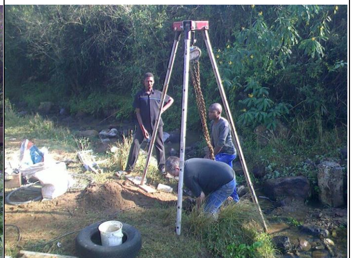
Fig. 3.6 Showing installation of a concrete lateral strut of the weir lintel into a hole by a friend helping. The strut was lowered in position by the large tripod shown that was made for the project by Michael Relihan.
