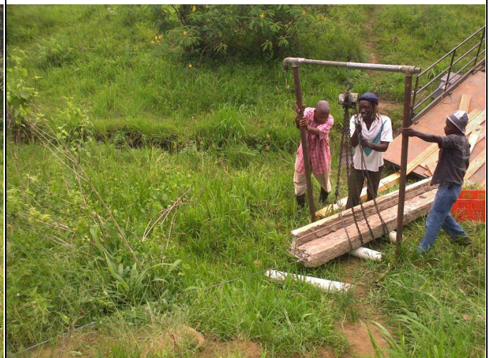
Fig. 3.4 Showing movement of the weir's lintel on rollers (previously garage door counter weights) by locals supported by a pipe scaffold and dragged by hand-operated winch attached to trees on the route.
