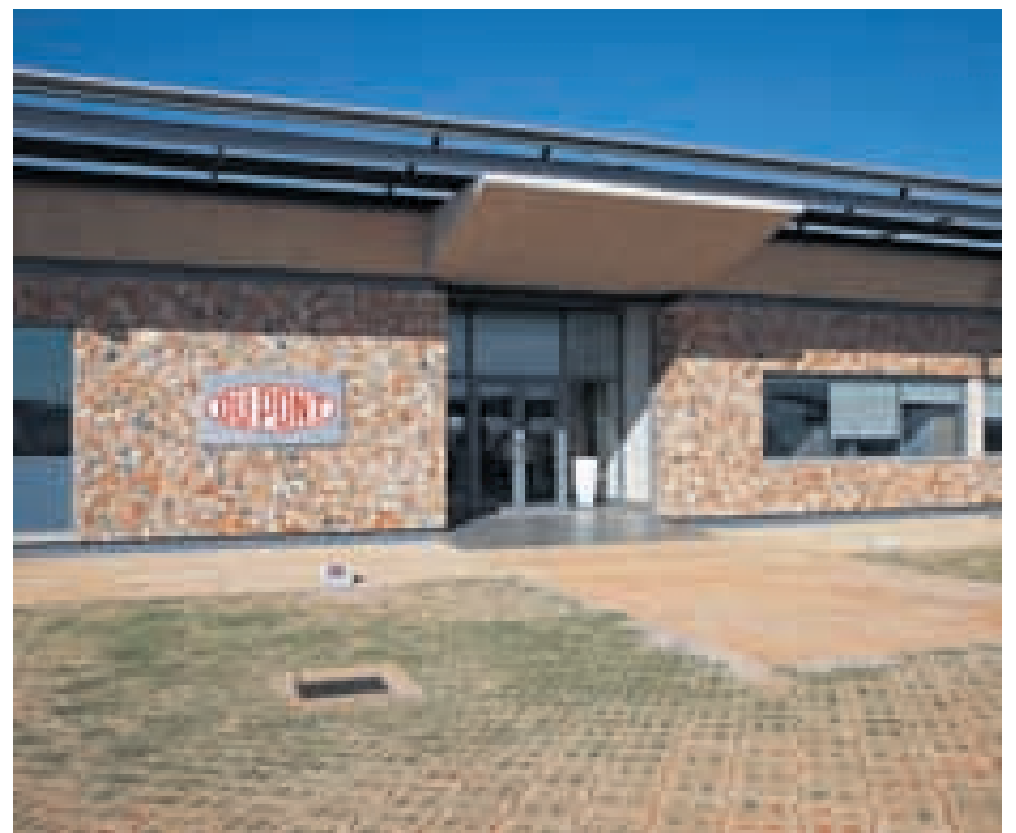
Du Pont's Africa regional technology centre in Delmas.
