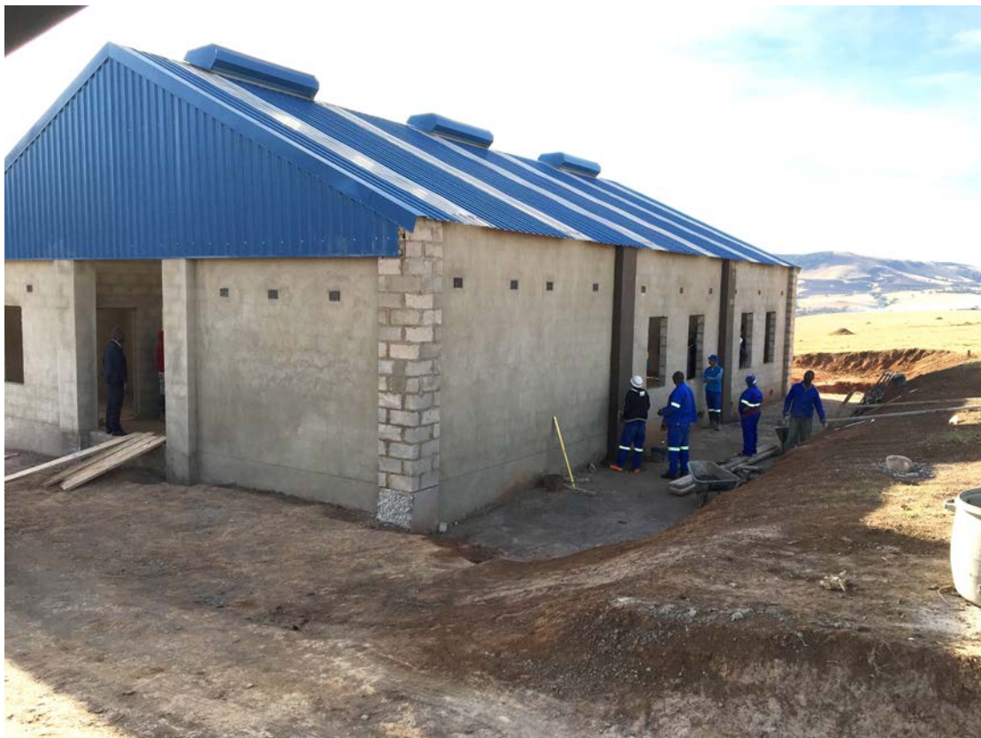
Exterior of the Glengary sheep shearing shed in uMzimkhulu
