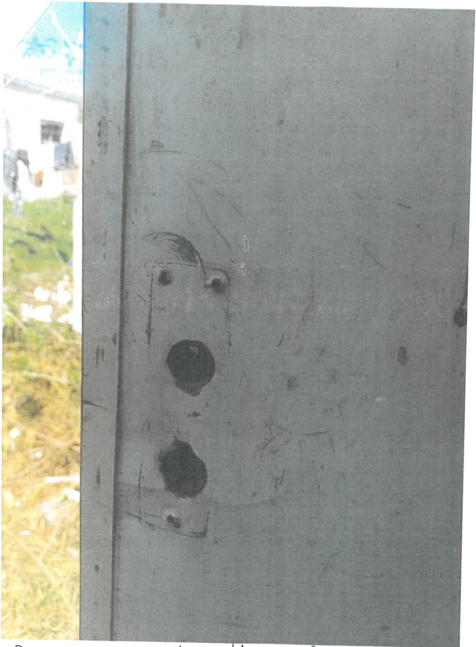
Door lock and handle replacement
