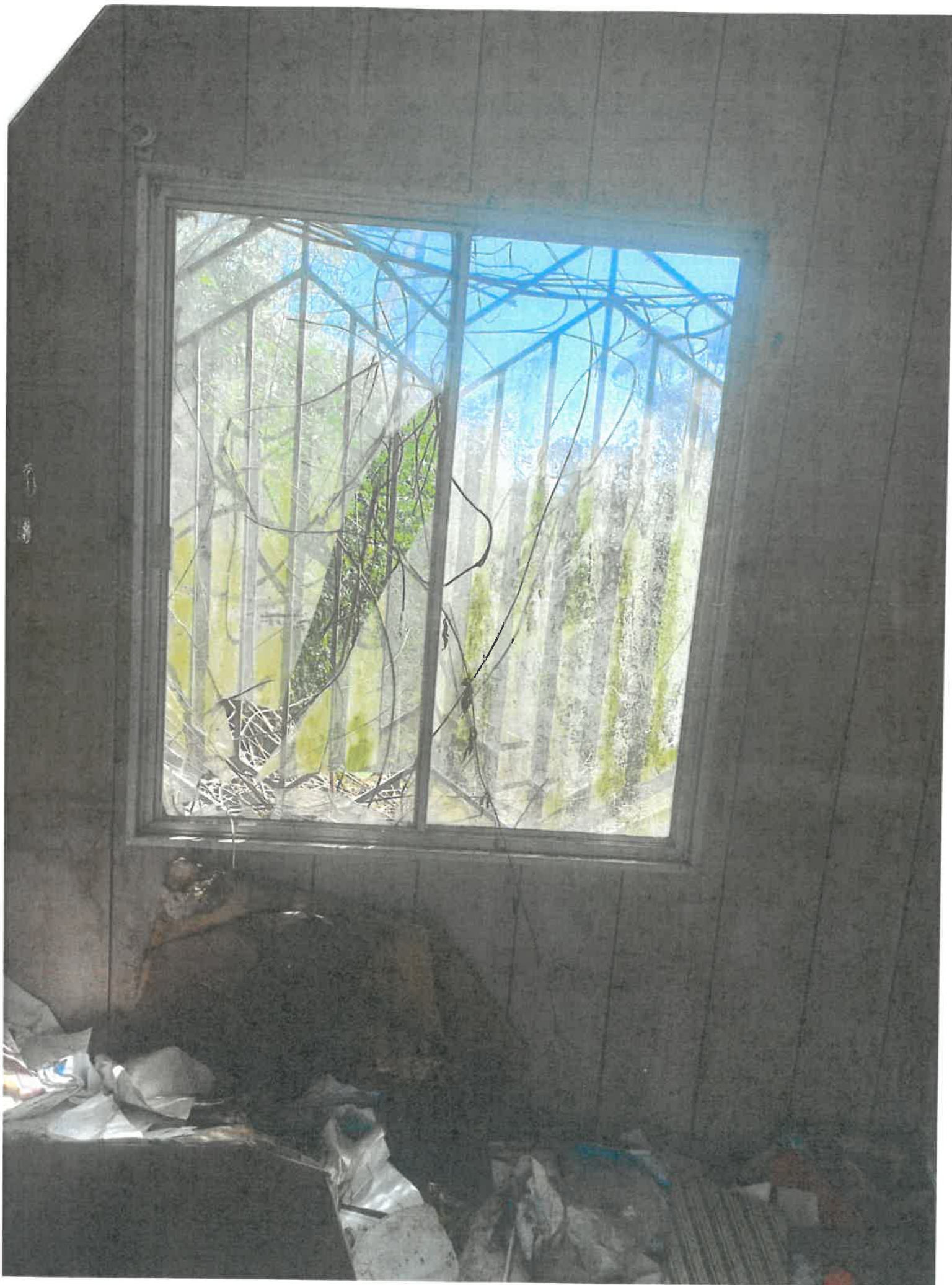
Broken window replacement
